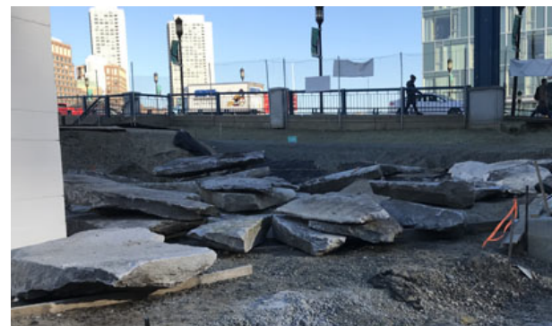
Granite on site
